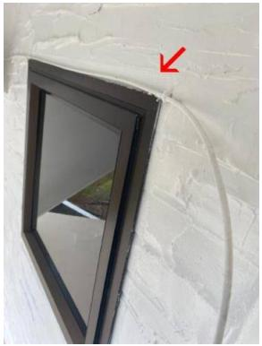
Joinery glazing rubbers have shrunk. Loose rubbers increase the risk of moisture ingress. We recommend engaging he services of a glazier to replace damaged rubbers to ensure glazing remains weathertight and secure.
