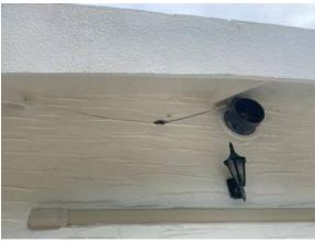
Redundant wiring to ceiling in garage. We recommend engaging the set of an electrician to inspect and isolate as required.
