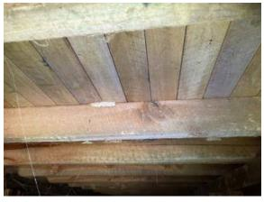
**Findings:** No Subfloor insulation present at the time of inspection. We recommend engaging the services of a insulation specialist to install subfloor insulation.
