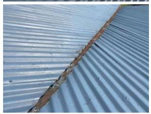
Numerous roof fixings have walked. These fixings will require tightening or replacement to ensure fixing penetrations remain watertight.
