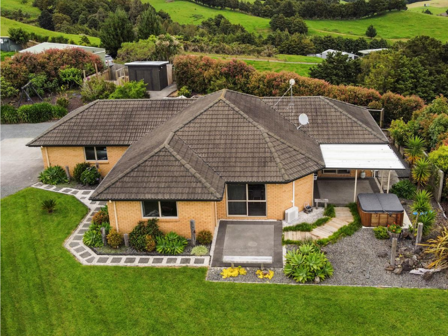
Ruatangata, 64 Crossett Road
