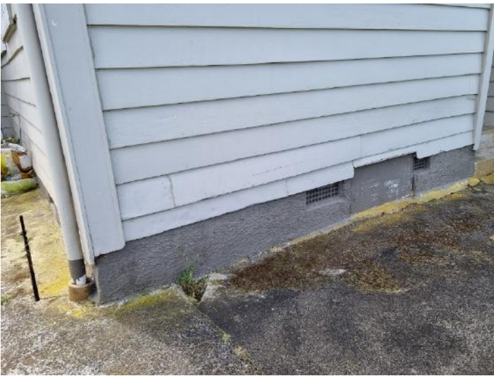
Weatherboard's showing signs of deterioration and recent unsatisfactory repairs have taken place, further investigation in places for repair
