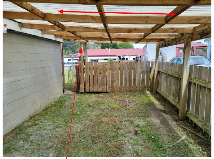
Carport rafters are sagging as the span is too much for the size of the timber. This is 100x50 and should be a minimum of 150x50
