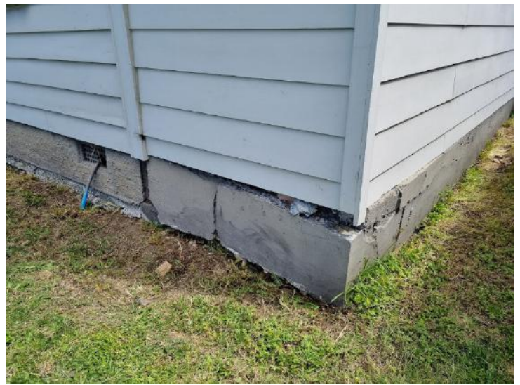
Weatherboard's showing signs of deterioration and recent unsatisfactory repairs have taken place, further investigation in places for repair
