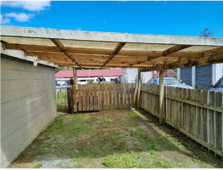
Carport rafters are sagging as the span is too much for the size of the timber. This is 100x50 and should be a minimum of 150x50
