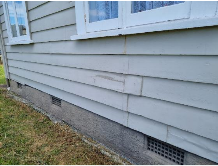
Weatherboard's showing signs of deterioration and recent unsatisfactory repairs have taken place, further investigation in places for repair
