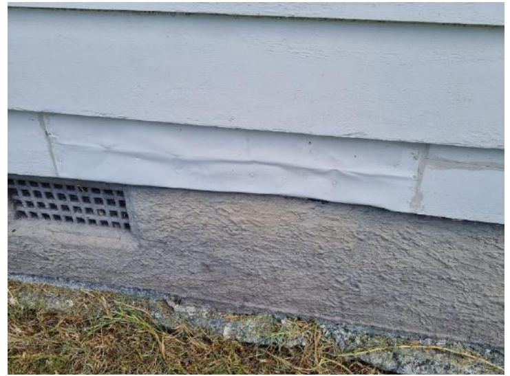
Weatherboard's showing signs of deterioration and recent unsatisfactory repairs have taken place, further investigation in places for repair
