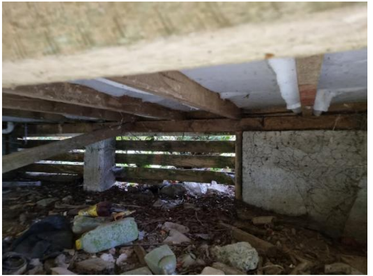
Sub structure framing looks reasonably sound with good air
