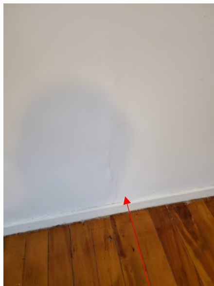
Possible historic water ingress in bedroom 1, issues present to the west wall
