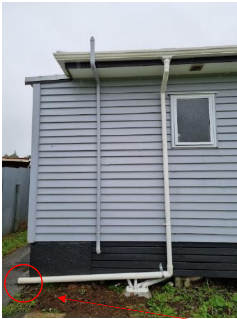
PVC downpipes pipe are not connected to any underground drainage – free flow over surface which does not comply with current NZ standards
