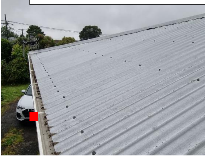
Roofing appears in good condition, estimate it has been replaced 5-10 years ago.
