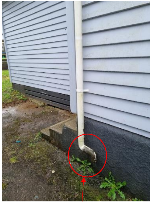
PVC downpipes pipe are not connected to any underground drainage – free flow over surface which does not comply with current NZ standards
