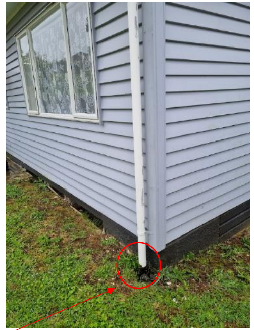
PVC downpipes pipe are not connected to any underground drainage – free flow over surface which does not comply with current NZ standards
