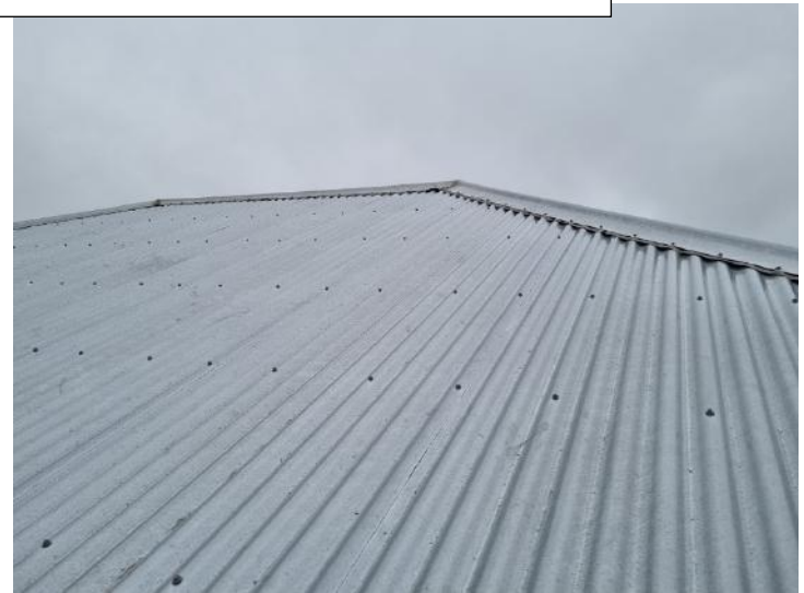
Roofing appears in good condition, estimate it has been replaced 5-10 years ago.
