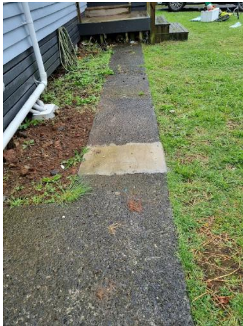
PVC downpipes pipe are not connected to any underground drainage – free flow over surface which does not comply with current NZ standards
