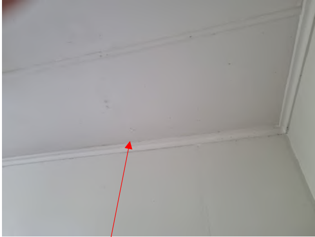
Signs of dampness to ceiling in bathroom
