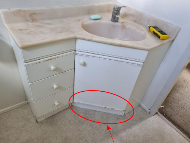
Water damage to vanity cabinetry
