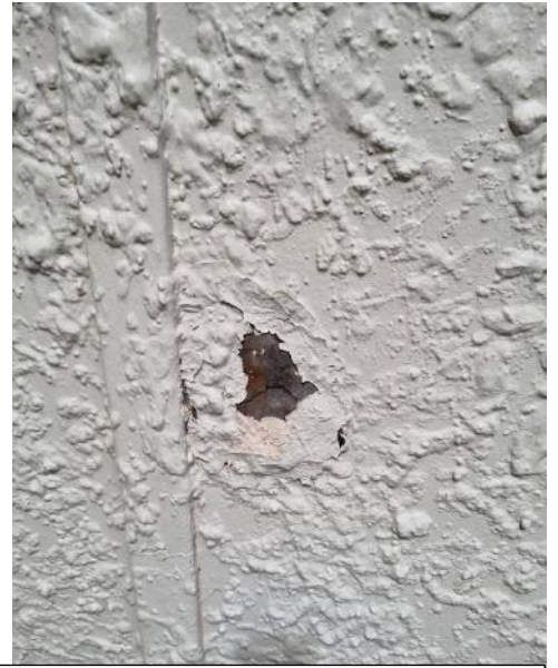
Hole on cladding vulnerable to water ingress
