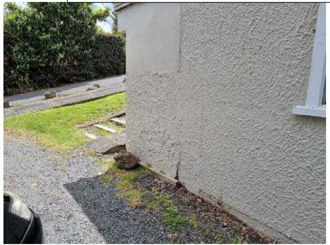
Hole on cladding vulnerable to water ingress
