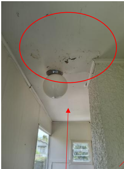
Ceiling water damage to laundry
