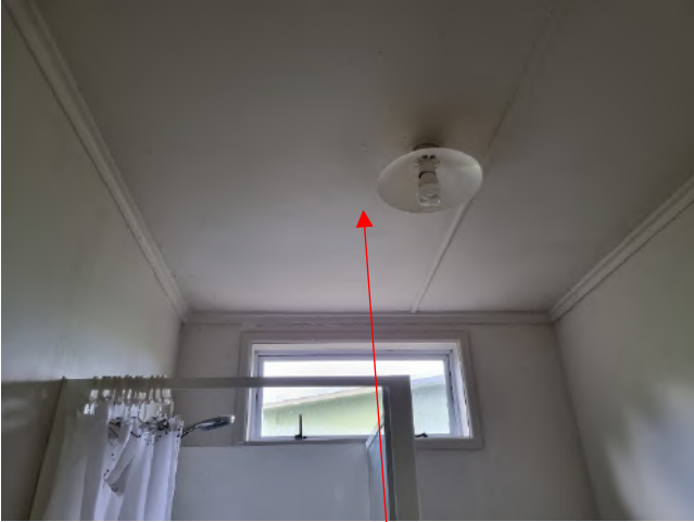
Signs of dampness to ceiling in bathroom
