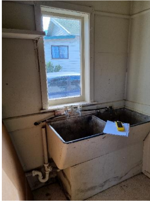
Moisture meter reading is greater than 80, this means material is at risk for wetness – further investigation is required
