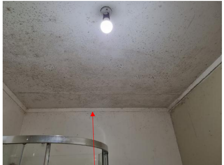
Bathroom has heavy signs of mould, most likely due to no extractor fan
