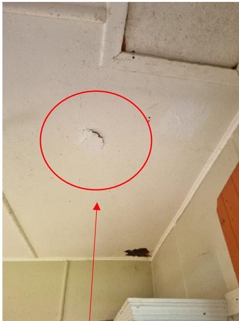
Damage to laundry ceiling - possible as a result from a past leak
