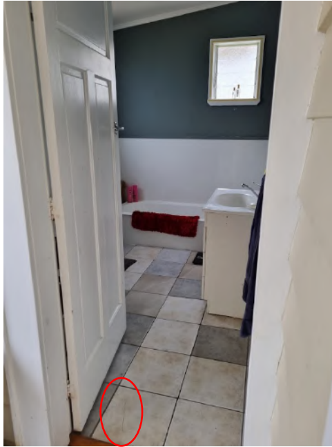
Tiles to floor in bathroom have a few broken that require replacing
