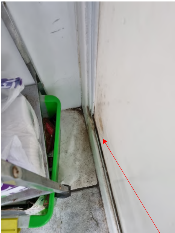
Left corner of shower lining needs repair
