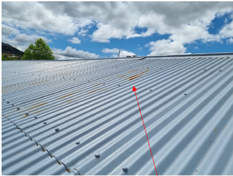
Roof is due for a replacement as it is showing signs of rust and deterioration
