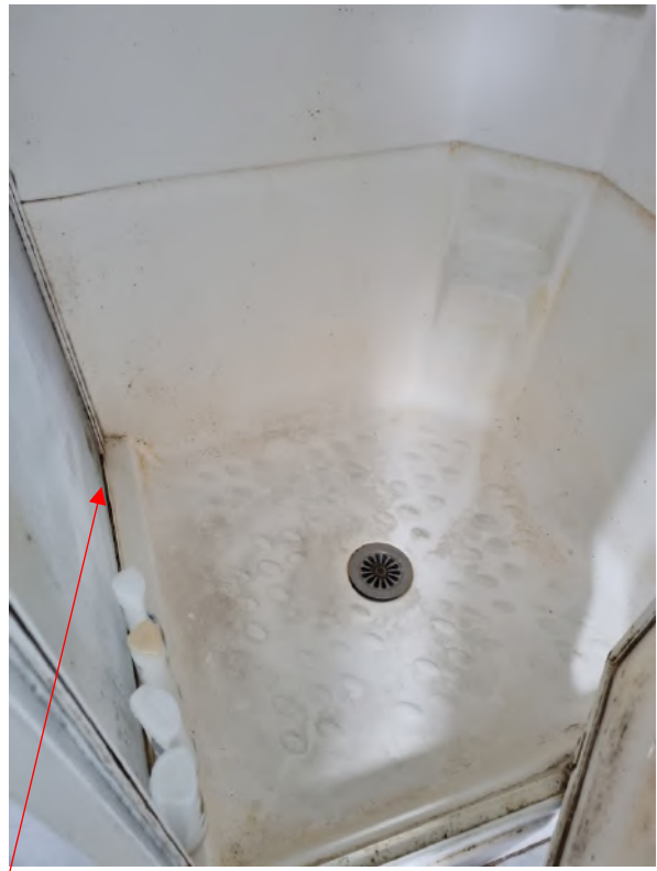
Moisture meter reading is higher than 80, this indicates great risk for wet material and further investigation is required
