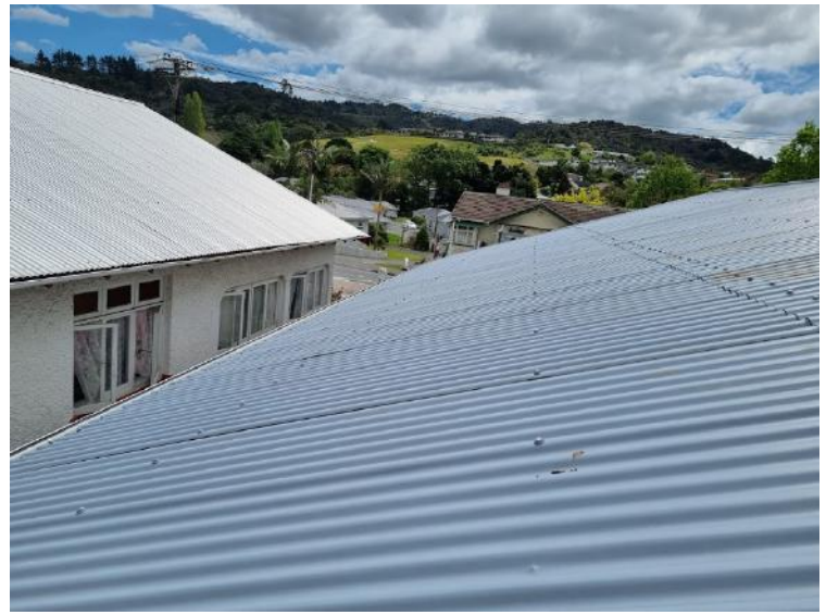
Roof is due for a replacement as it is showing signs of rust and deterioration
