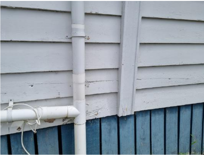
Signs of deterioration to the tongue and groove soffit boards, the timber cladding, the window facings, and corner facings
