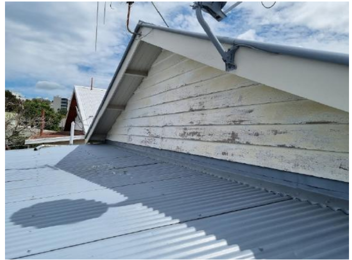
Exterior cladding would benefit with a complete paint
