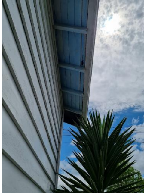
Signs of deterioration to the tongue and groove soffit boards, the timber cladding, the window facings, and corner facings
