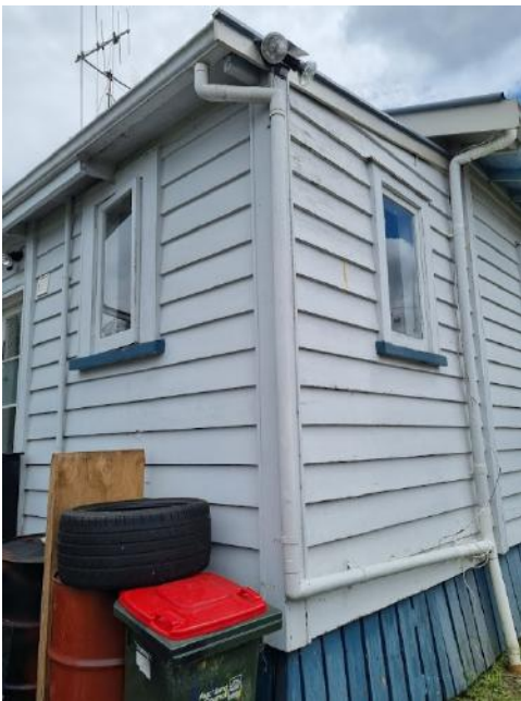
Signs of deterioration to the tongue and groove soffit boards, the timber cladding, the window facings, and corner facings
