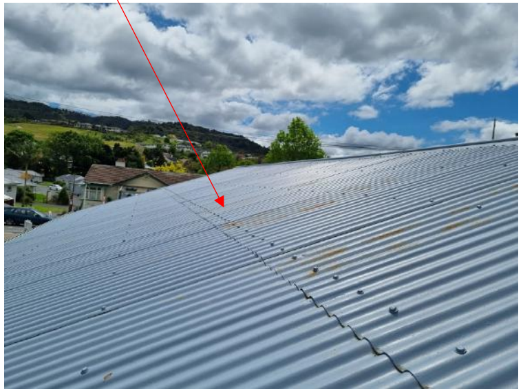
Roof is due for a replacement as it is showing signs of rust and deterioration
