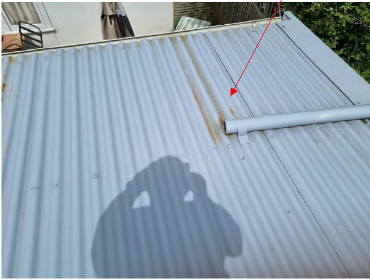
Roof is due for a replacement as it is showing signs of rust and deterioration
