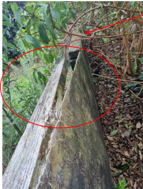
Plywood fence at rare needs maintenance
