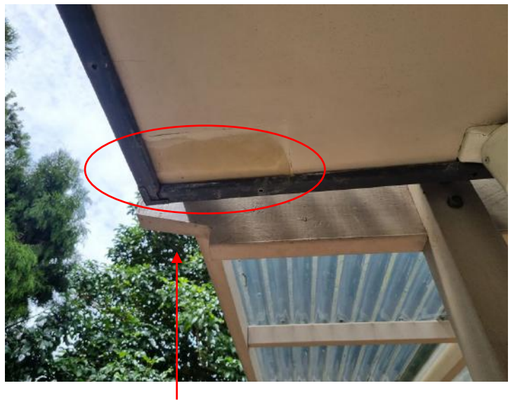
Small patch job has been done in corner of roof.
