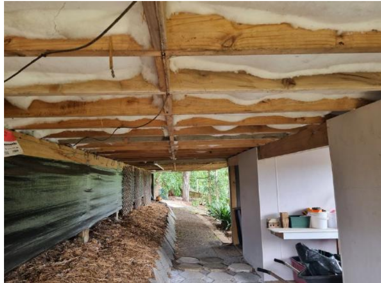
2x sheds under house were dry. Both are part board flooring and lined with fibrolite cladding.
