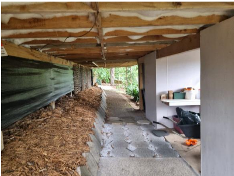
2x sheds under house were dry. Both are part board flooring and lined with fibrolite cladding.
