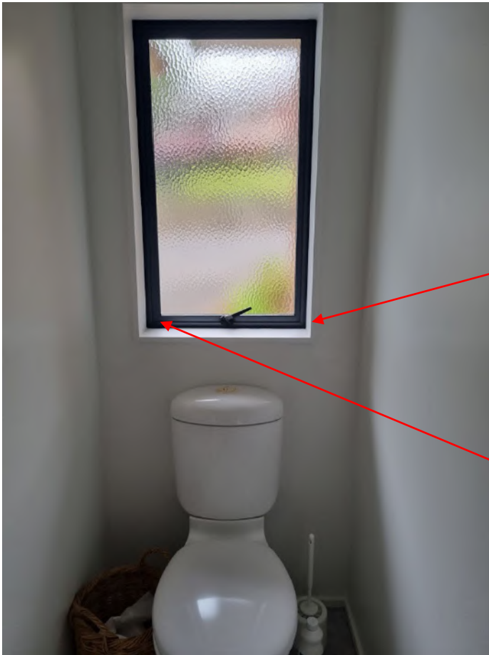
Separate toilet has no vent
