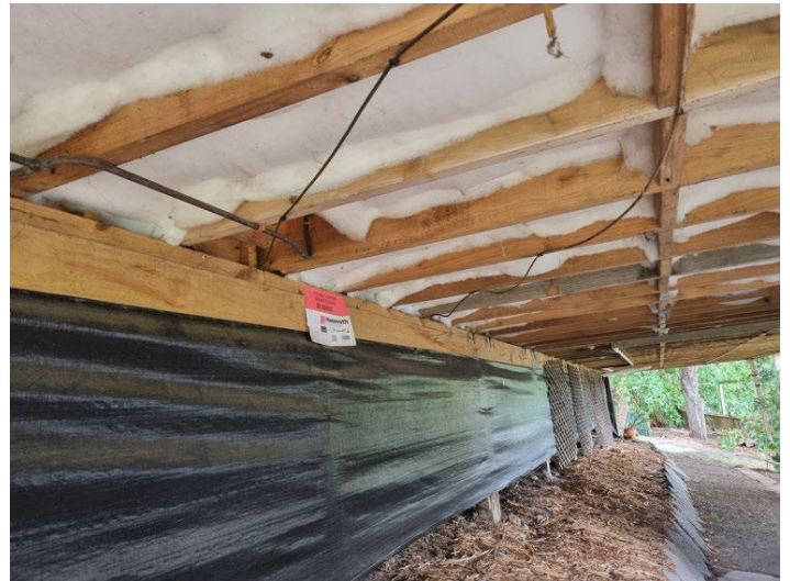
2x sheds under house were dry. Both are part board flooring and lined with fibrolite cladding.
