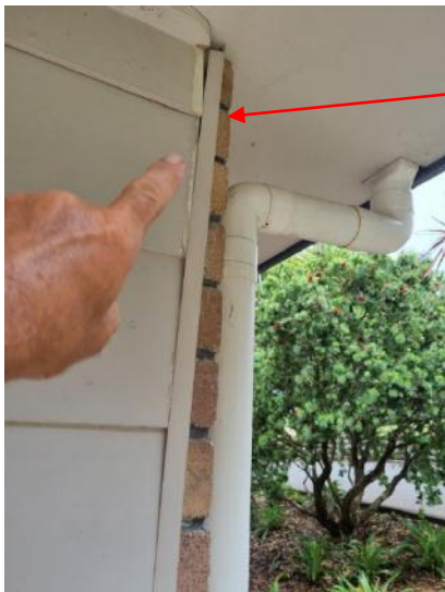
Corner joint (PVC capping) needs to be refitted.
