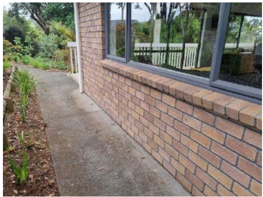
Corner joint (PVC capping) needs to be refitted.
