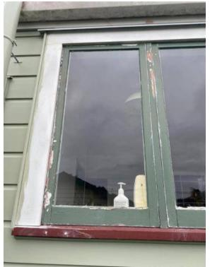
Loose glazing putty to window joinery. We recommend replacing compromised putty to ensure window panes remain glazing remains secure and weathertight.
