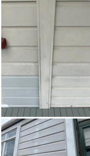
Weatherboard have been primed but require top coat, paint lift to original weatherboards. Weatherboards will require appropriate preparation and paint to ensure cladding remains well sealed. Failure to maintain paint coating increases the risk of exposure
