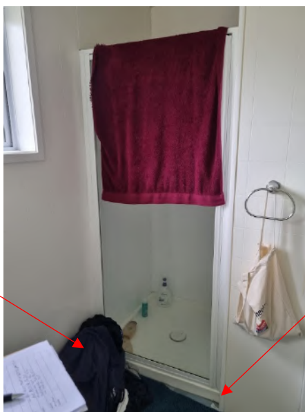
Moisture meter readings are higher than 80, this indicates there is wet materials and is at risk. Further investigation is required
