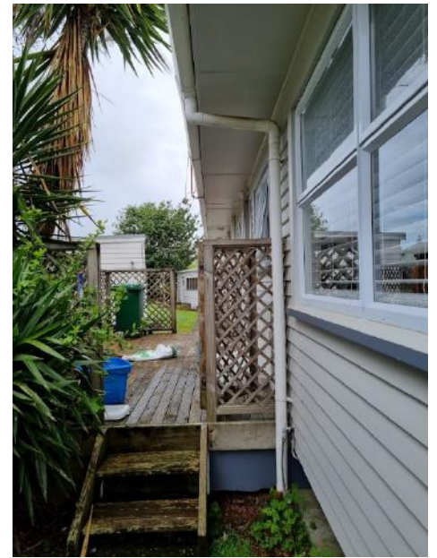
Timber decking to the back of the property is in poor condition – could do with replacing as rotting in places
