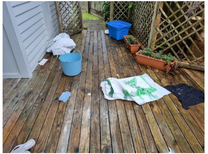
Timber decking to the back of the property is in poor condition – could do with replacing as rotting in places
