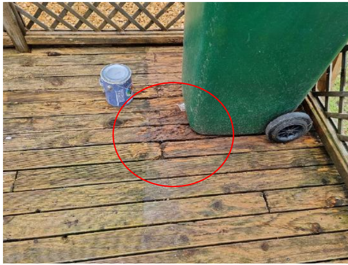
Timber decking to the back of the property is in poor condition – could do with replacing as rotting in places
