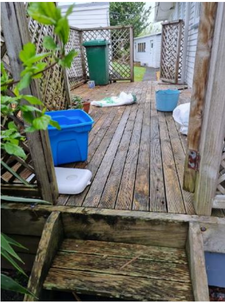
Timber decking to the back of the property is in poor condition – could do with replacing as rotting in places
