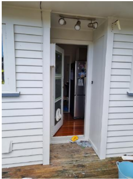
Timber decking to the back of the property is in poor condition – could do with replacing as rotting in places
