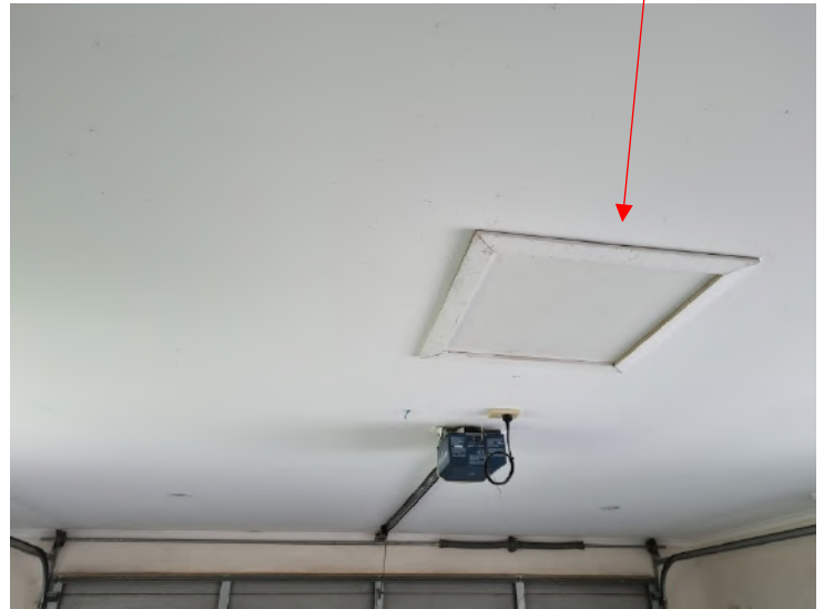
Roof hatch surround in garage requires re-fixing
