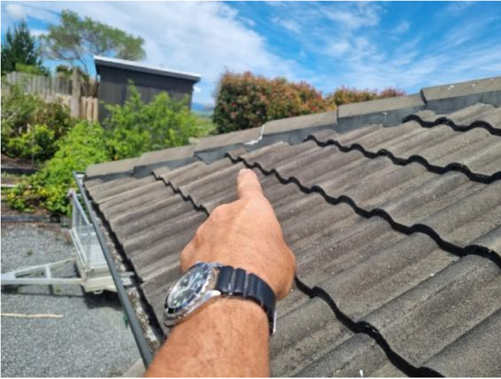
Concrete tile roof at ridges plaster work needs to be sealed to prevent water ingress. Appears in reasonable condition
