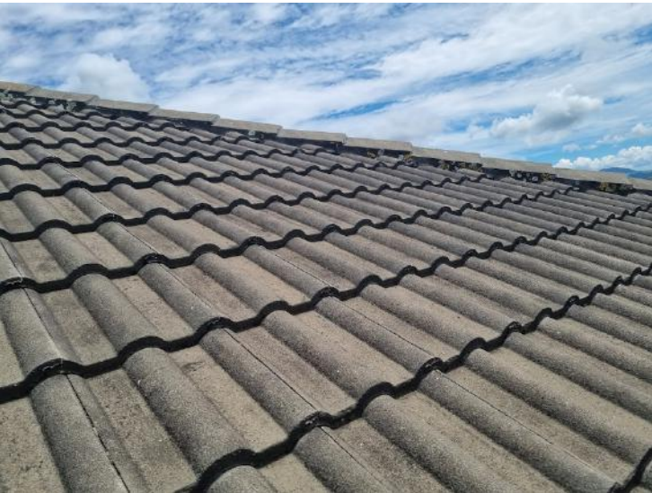
Concrete tile roof at ridges plaster work needs to be sealed to prevent water ingress. Appears in reasonable condition
