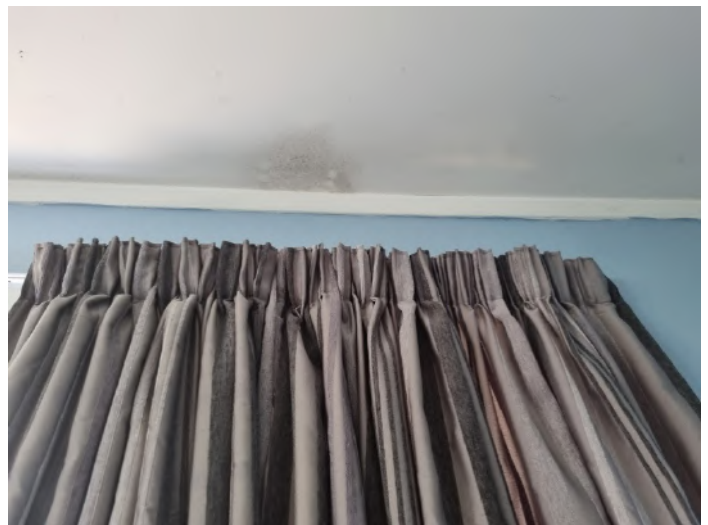
Patch of mould present to right hand side of main window in bedroom 3 (Master). Moisture reading is 4.5 and is not showing any signs of damp.
