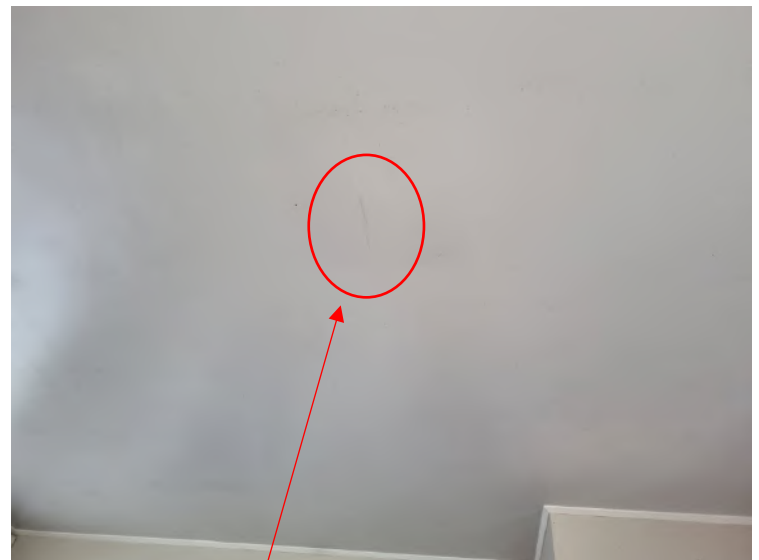
Crack in the lounge ceiling where it shows slight sagging, unable to obtain a moisture reading. Could be a result for several reasons, it does appear dry at this point.
