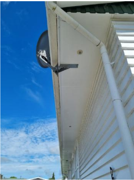
Fibrolite will most likely contain asbestos, present to the base, gable, and entryway
