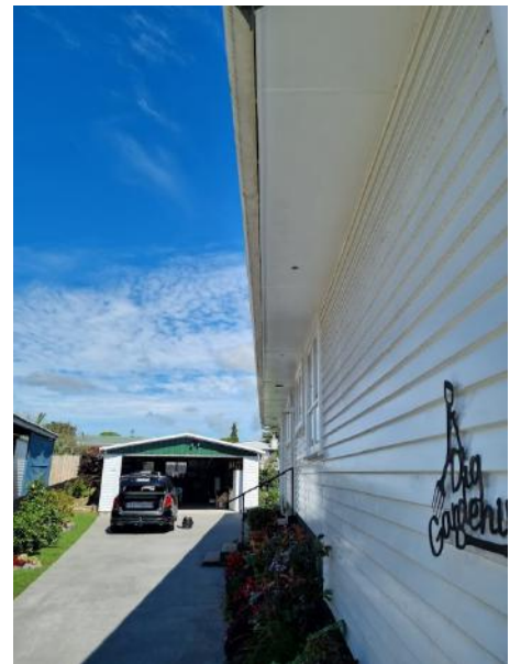
Fibrolite will most likely contain asbestos, present to the base, gable, and entryway
