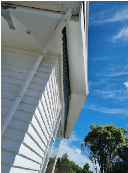
Fibrolite will most likely contain asbestos, present to the base, gable, and entryway
