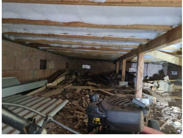
Subfloor structure appears sound
