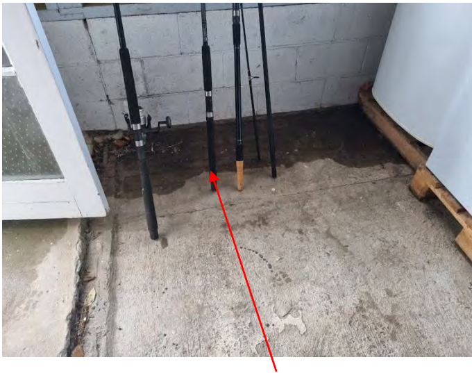
Garage showing signs of water ingress when it rains to the concrete floor.
