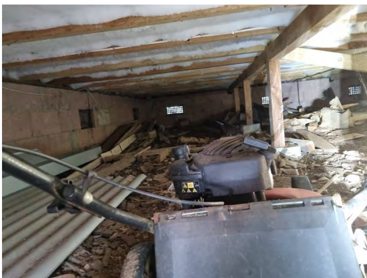
Subfloor structure appears sound
