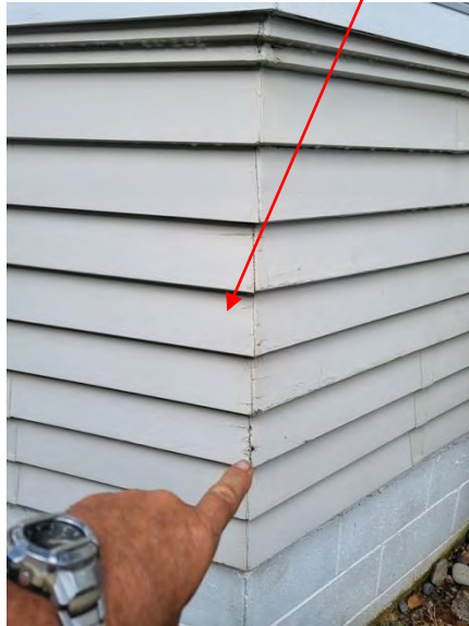
Sunroom side of the house has some rotten timber boards
