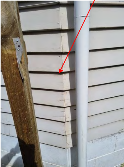
Sunroom side of the house has some rotten timber boards
