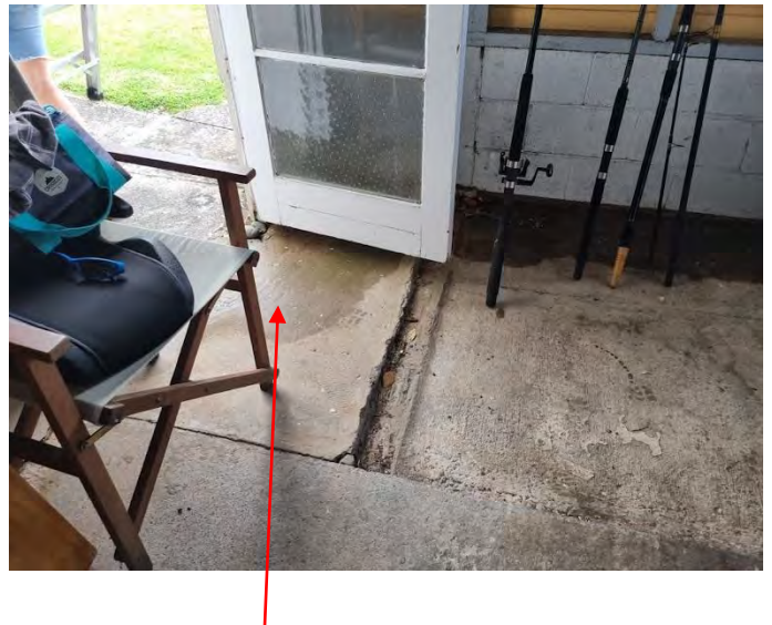
Garage showing signs of water ingress when it rains to the concrete floor.
