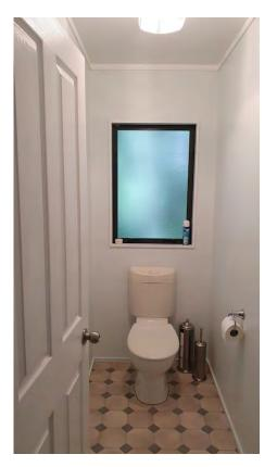
Separate window requires security stays to protect from falling- a simple fix for a builder or Aluminium joiner to comply with today's building standards
