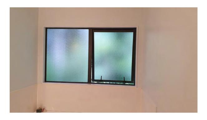
Main bathroom window requires security stays to protect from falling- a simple fix for a builder or Aluminium joiner to comply with today's building standards
