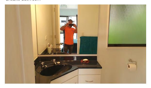
Ensuite window requires security stays to protect from falling- a simple fix for a builder or Aluminium joiner to comply with today's building standards
