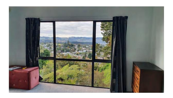
Master bedroom window: Under current building requirements, this glass would be safety glass. Recommendation is to swap out and replace the existing glass panel to safety glass.
