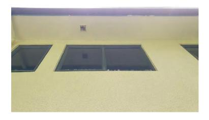
Insuclad does not sit on a cavity. This is how these homes were built late 90s early 2000s. Current standards, you would have a cavity. Visually, I cannot see any problems with moisture ingress.
