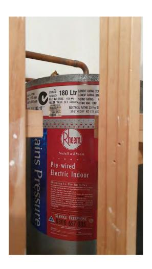
For best practice, hot water cylinder should be on a tray in case it ever leaks
