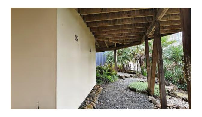
Deck posts to rear have twisted and recommend replacing.
